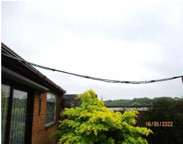
View from rear elevation to neighbouring boundary (no. 54).
