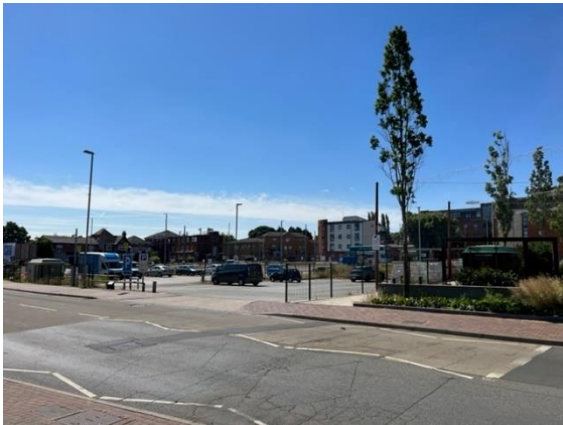
View of existing site access
