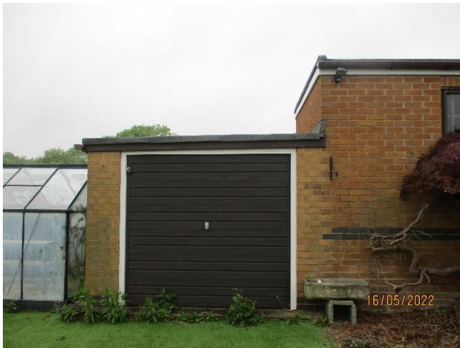
Garage/ outbuilding on boundary with no. 50.
