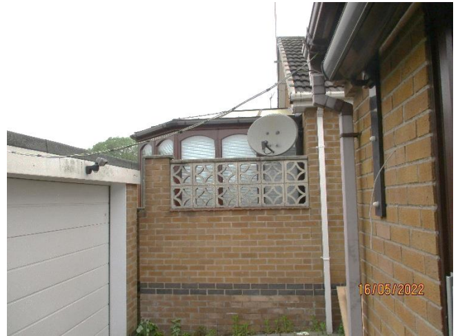
View from rear elevation to neighbouring boundary (no. 50).
